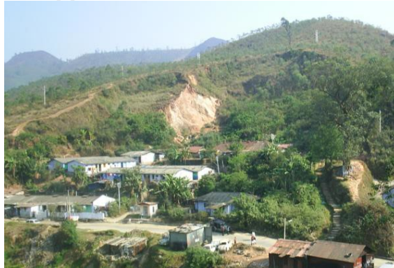
Figure 7. Anthoniar Colony Landslide
