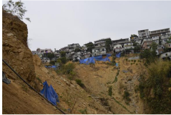
Figure 5. Landslide at Ramhlun Sports Complex
