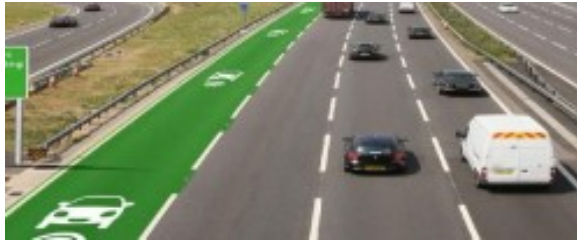
Fig1 A practical example of wireless charging of lane in UK.
