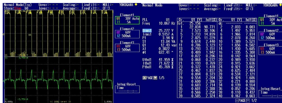
Figure.13. Power Analyzer results of Nine Phase Induction Motor Drive for 10 Hz
